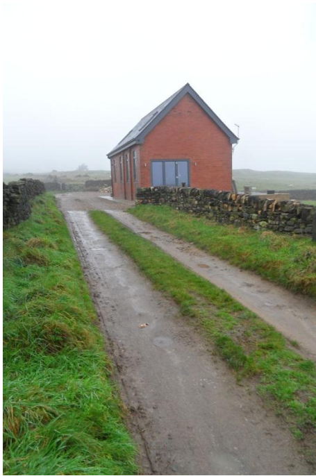
Photo 3.7: Redeveloped Pump House, Occupation Lane
